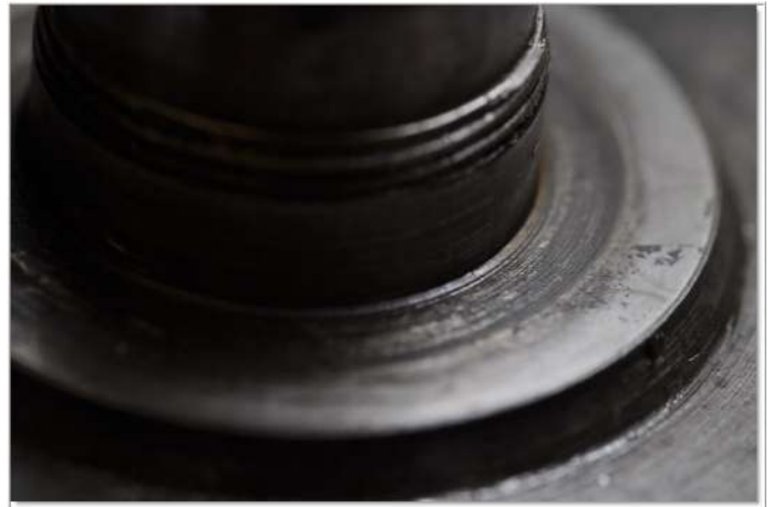
Inner wall for rollers with main bearing ring removed, showing slight clean up of wall above diameter of main bearing inner ring that had been ground in situ.
